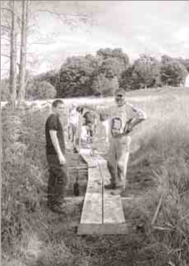
Howie Kargman and other Fellowship members installed a puncheon over a wet section of trail at Mobbs Valley in Jericho in September 2008. PHOTO BY BROOKE SCATCHARD.
