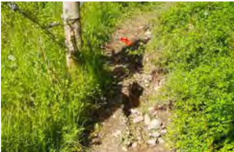
Erosion on the Russell Trail.
