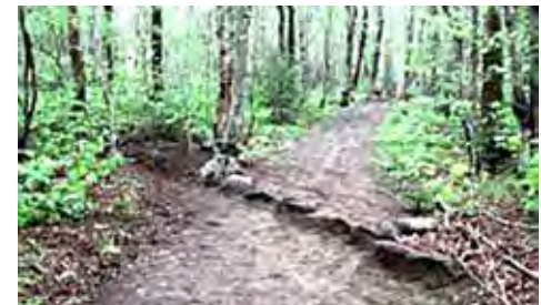
Water bar in place.
