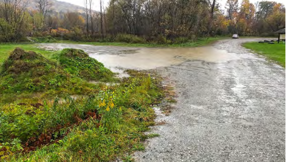
Starksboro Cota Ballfields and parking lot are inundated during a rain storm. Photo credit: Chris Runcie
