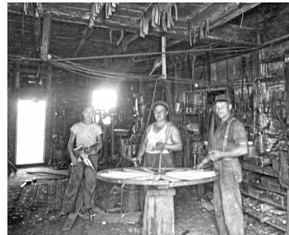
J.P., center, and Vic, left, repairing wagon wheel 1939
