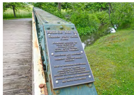
Button head rivets hold Hinesburg truss bridge together.
