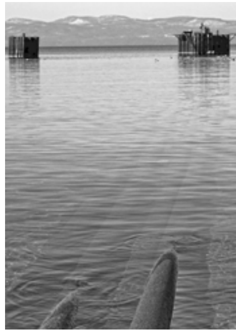
Two Texaco Beach Oil Dolphins and Underwater Lines Reaching Shore.
