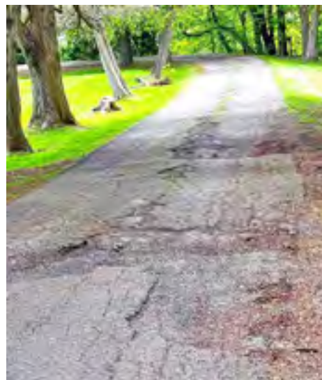
Roads need to be maintained and ditched to manage stormwater, trees need to be trimmed or felled, and many stones need repair or resetting.
