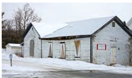
The old Vestry building next to St. Jude’s will be dismantled.
